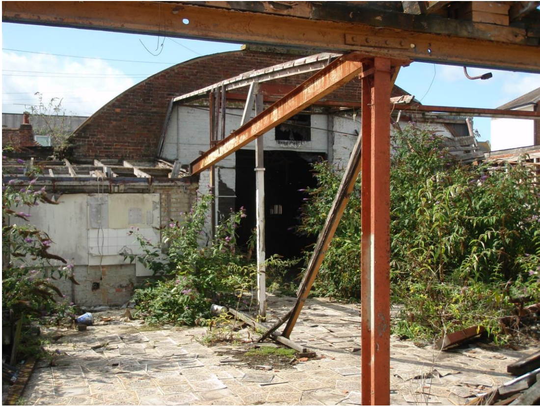
Plate 13. Demolished rear of building (looking South)
