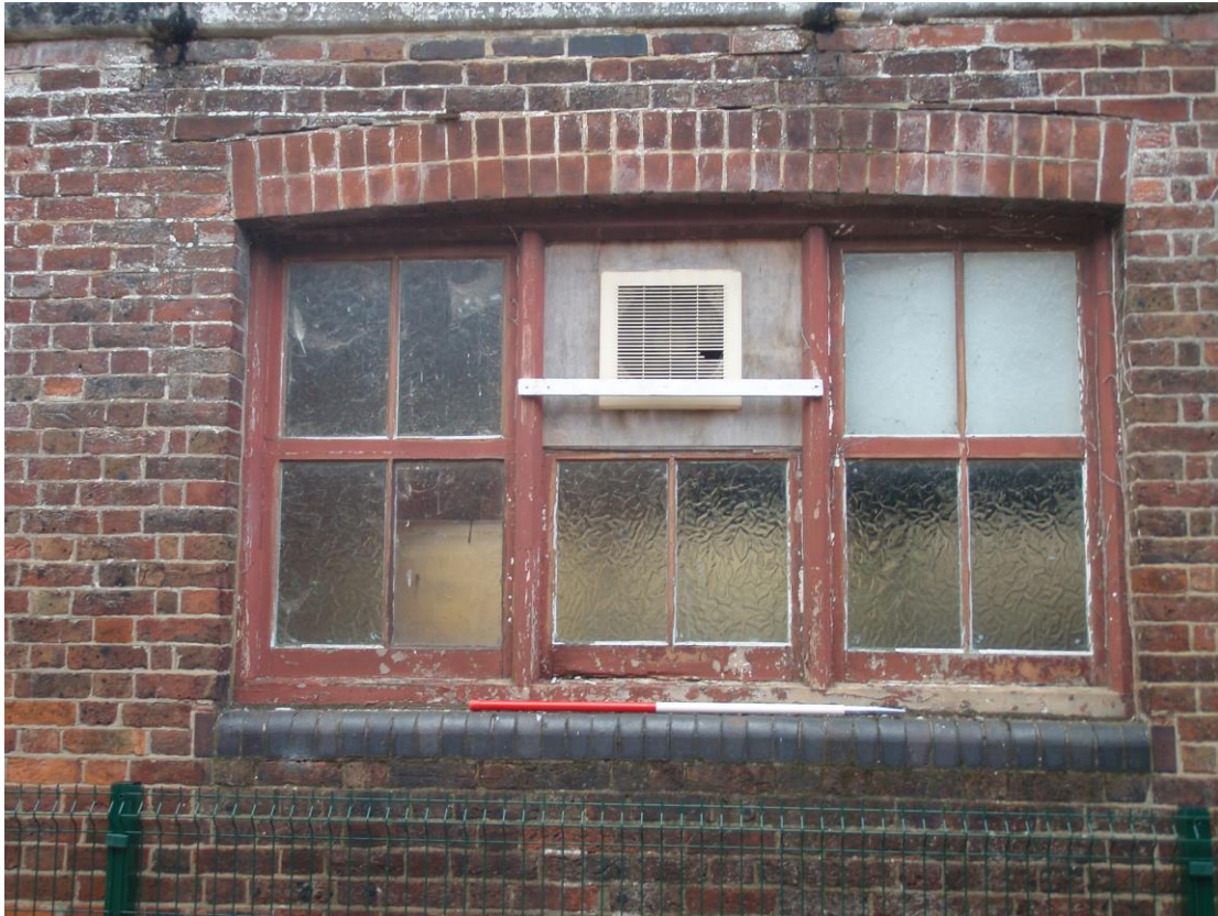
Plate 11. Detail of external west wall windows of main building (looking East 1m scale)
