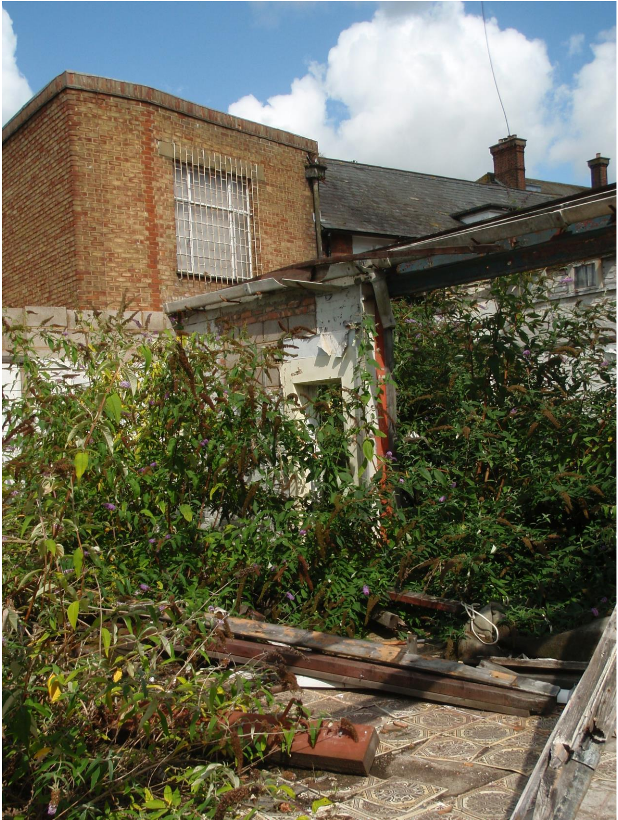
Plate 6. Demolished building at rear of premises (looking South)
