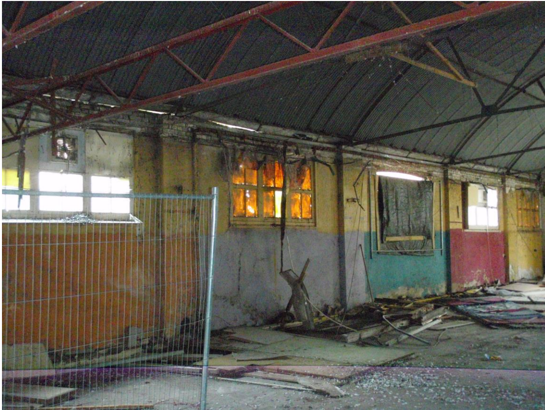
Plate 9. West wall of main building (looking North 2m scale)
