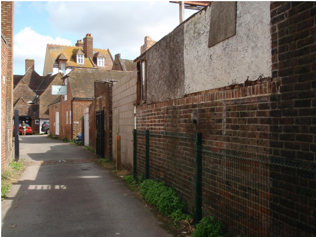
Plate 12. External west wall of main building (looking North)
