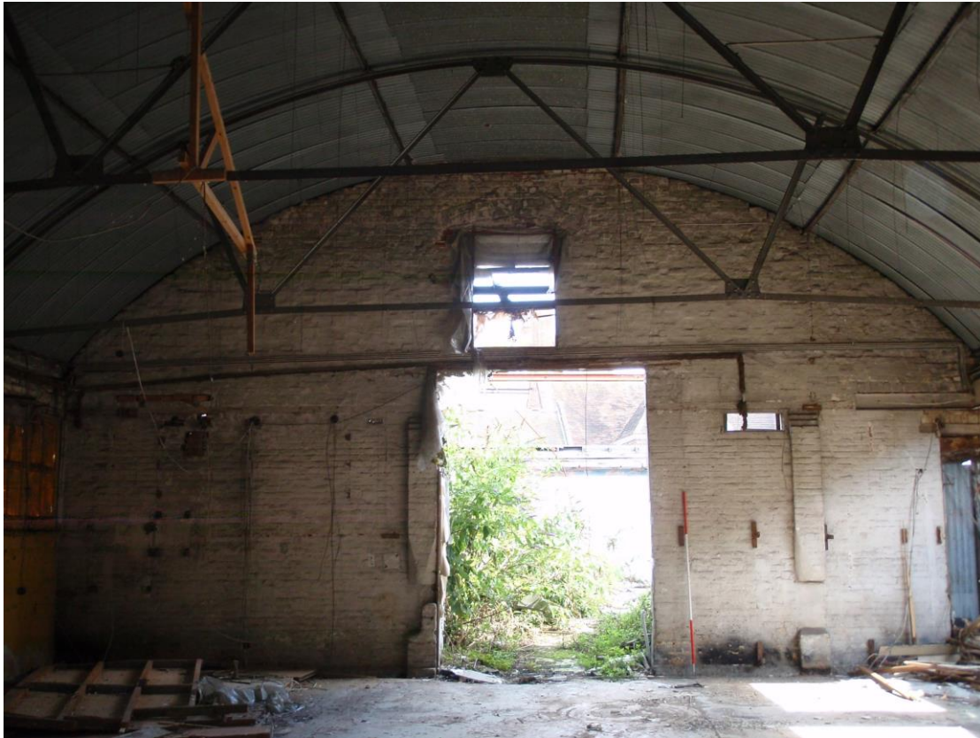
Plate 7. Rear wall of main building (looking North 2m scale)
