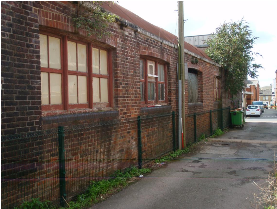
Plate 10. External west wall of main building (looking South 1m scale)
