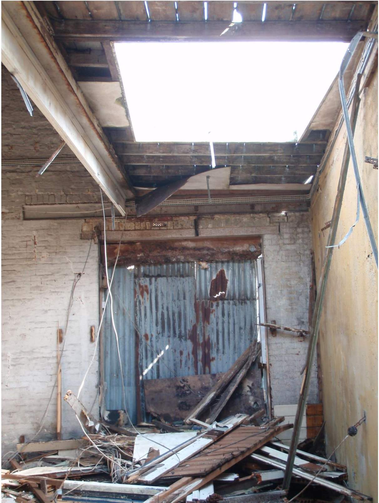
Plate 5. Interior of rear of building (looking North)
