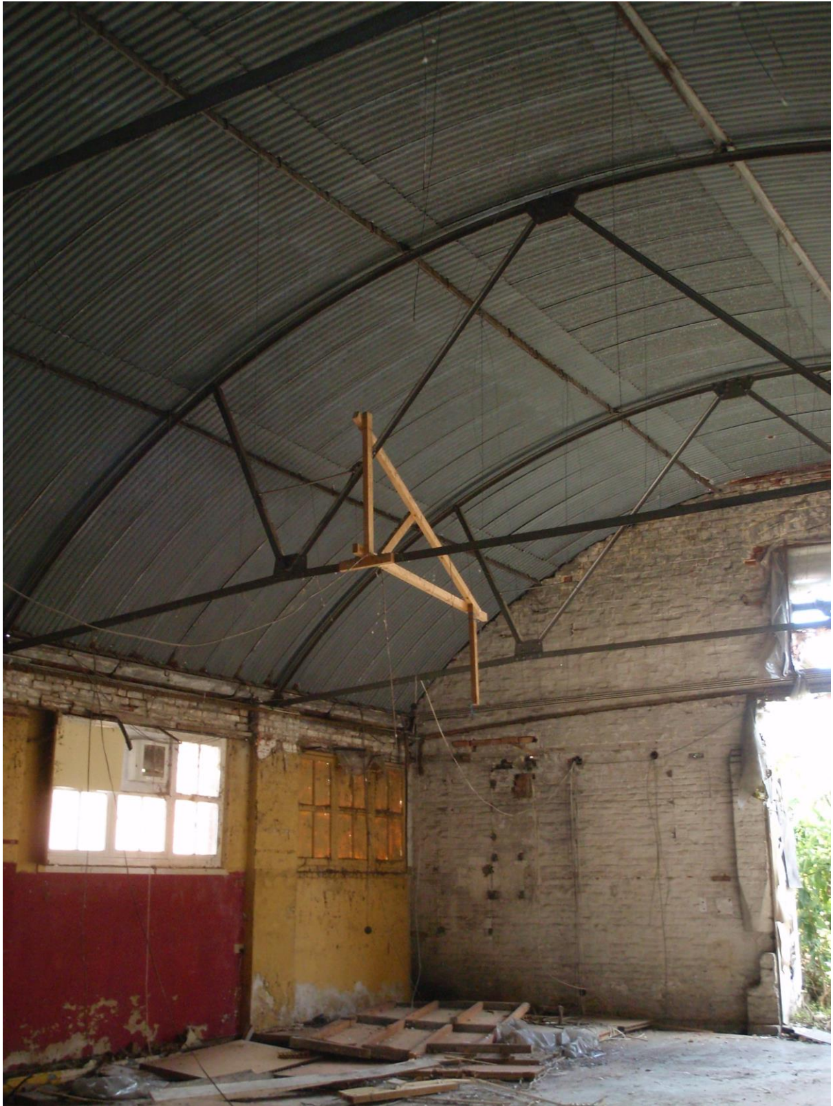
Plate 3. Interior of rear of building (looking North)
