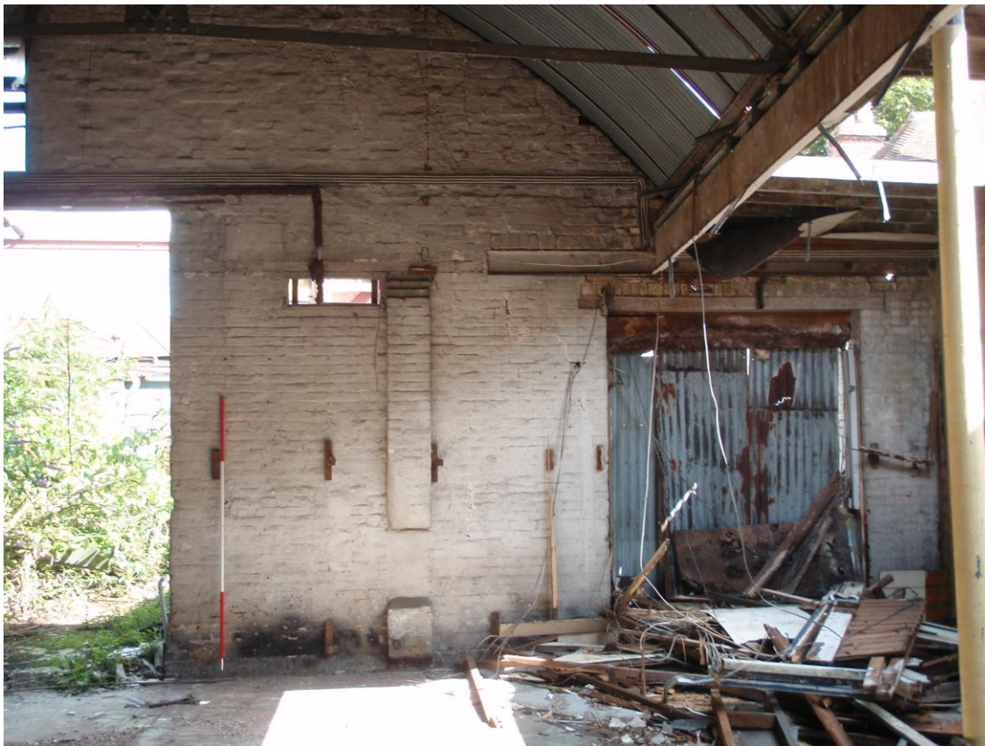
Plate 8. Rear wall of main building (looking North 2m scale)
