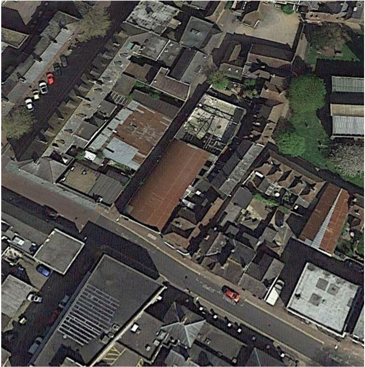
AP 2. 2017 showing demolition to rear of the PDA
