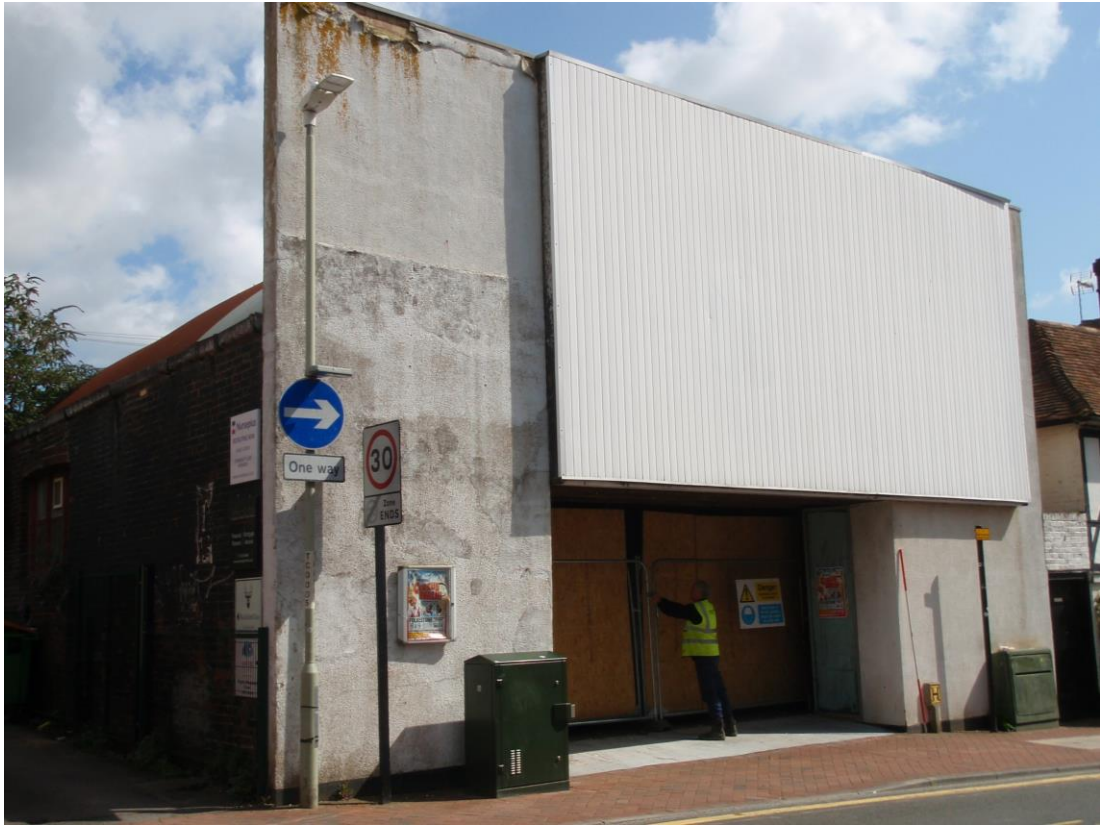
Plate 15. Frontage of main building (looking NE 2m scale)
