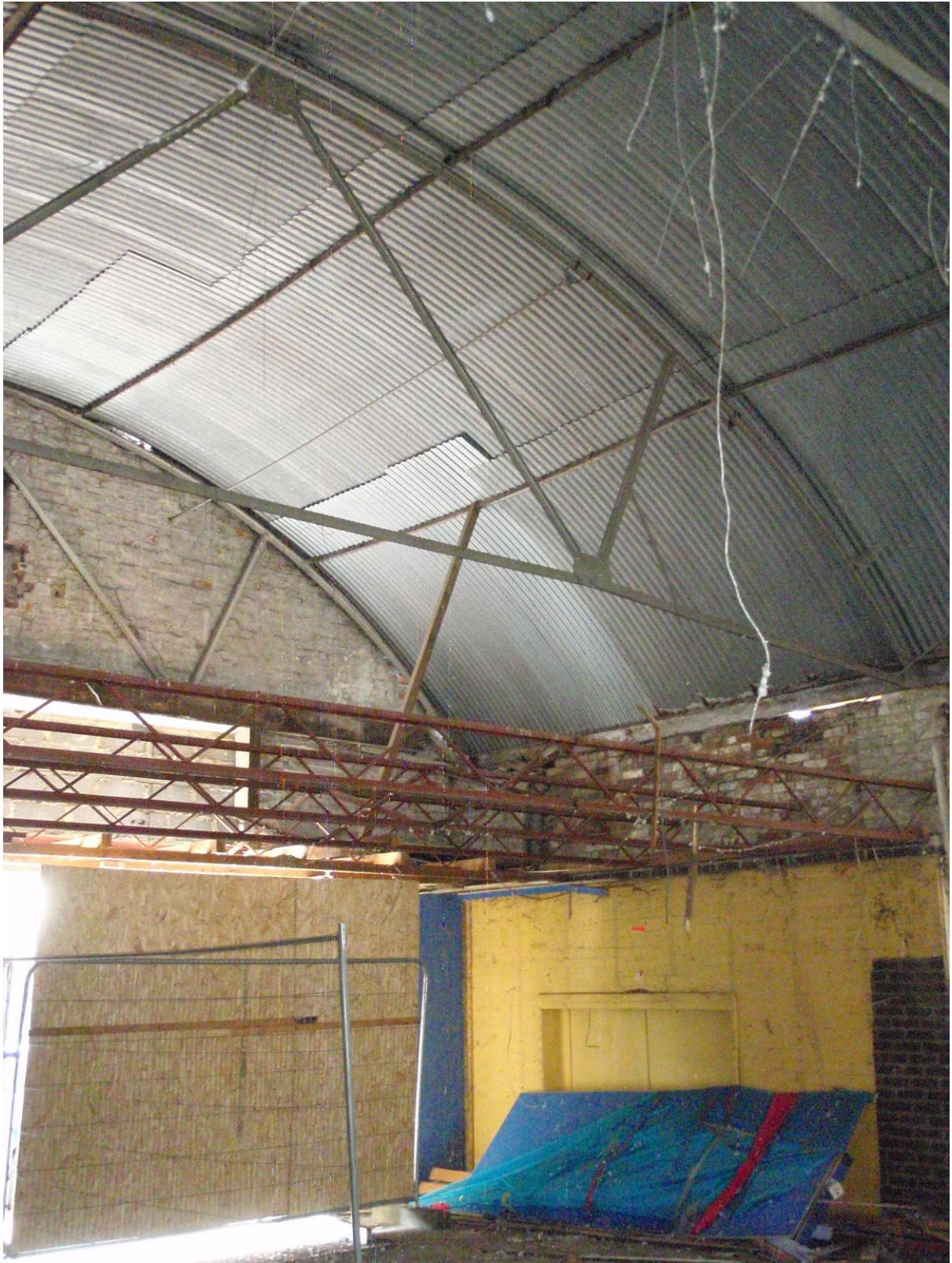
Plate 4. Interior of building (looking NE)
