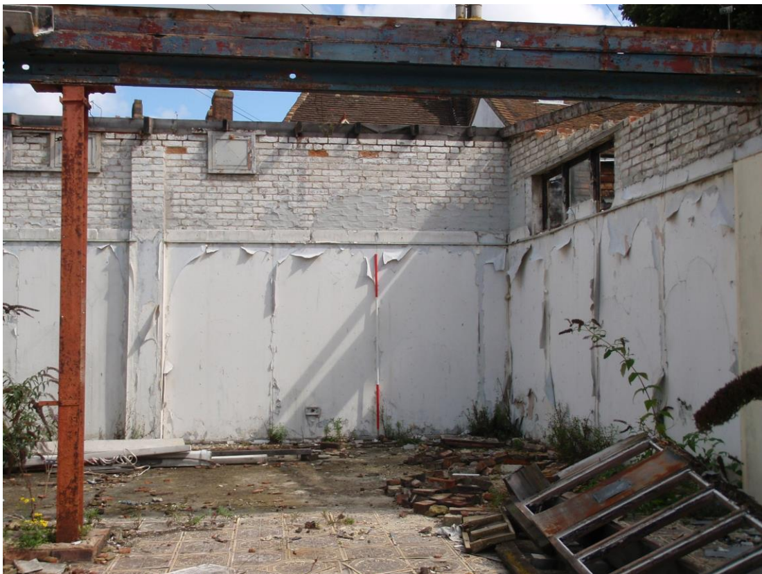
Plate 14. Demolished rear of building (looking north)
